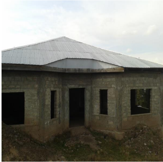
Front view of under construction Cafeteria
