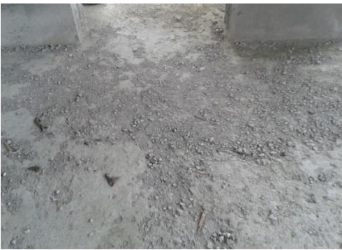
Damaged PCC Flooring indicative of poor quality of concrete used
