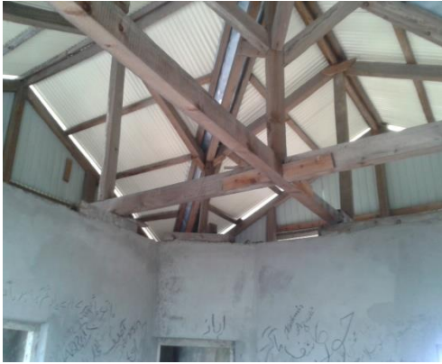
Wooden Trusses without any properly spaced Vertical Members
