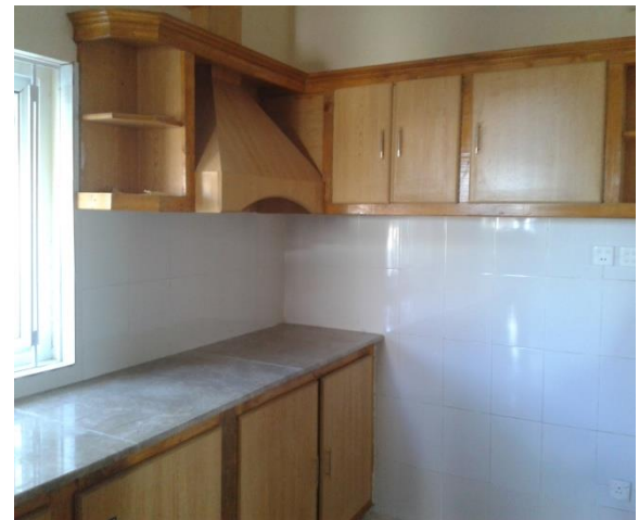
Kitchen of New Rest House
