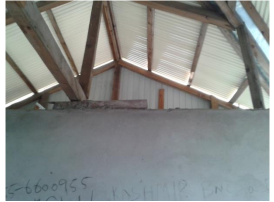
Wooden Trusses without any properly spaced Vertical Members
