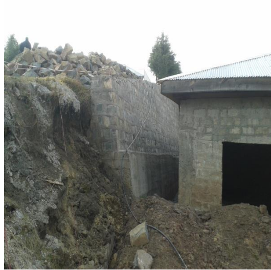
Retaining Wall constructed by PWD
