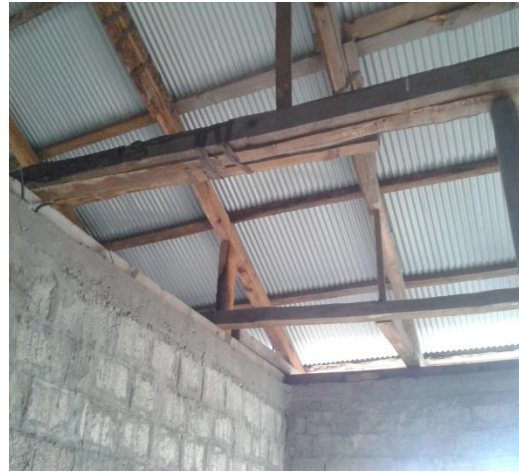
Horizontal wooden member supported by iron Vertical strips
