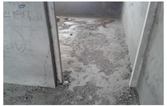
Damaged PCC Flooring indicative of poor quality of concrete used
