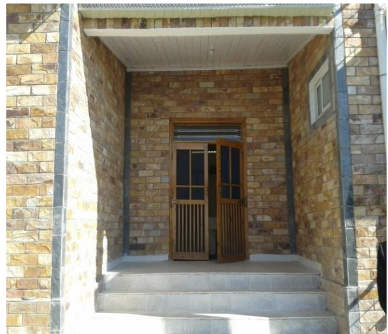
Entrance of New Rest House Building
