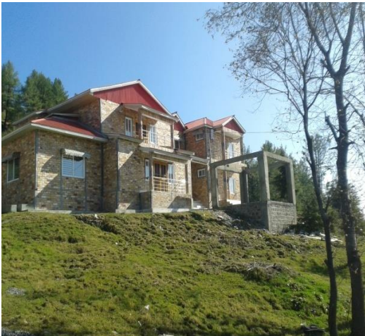
View of Rest House Building
