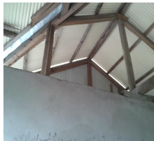
Construction of Trusses has been done without following engineering design/standards.
